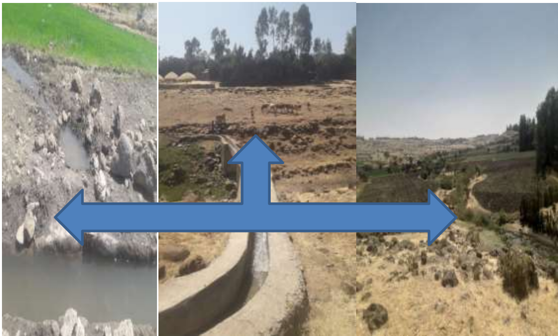
Figure 7.3: Water losses from the main canal
