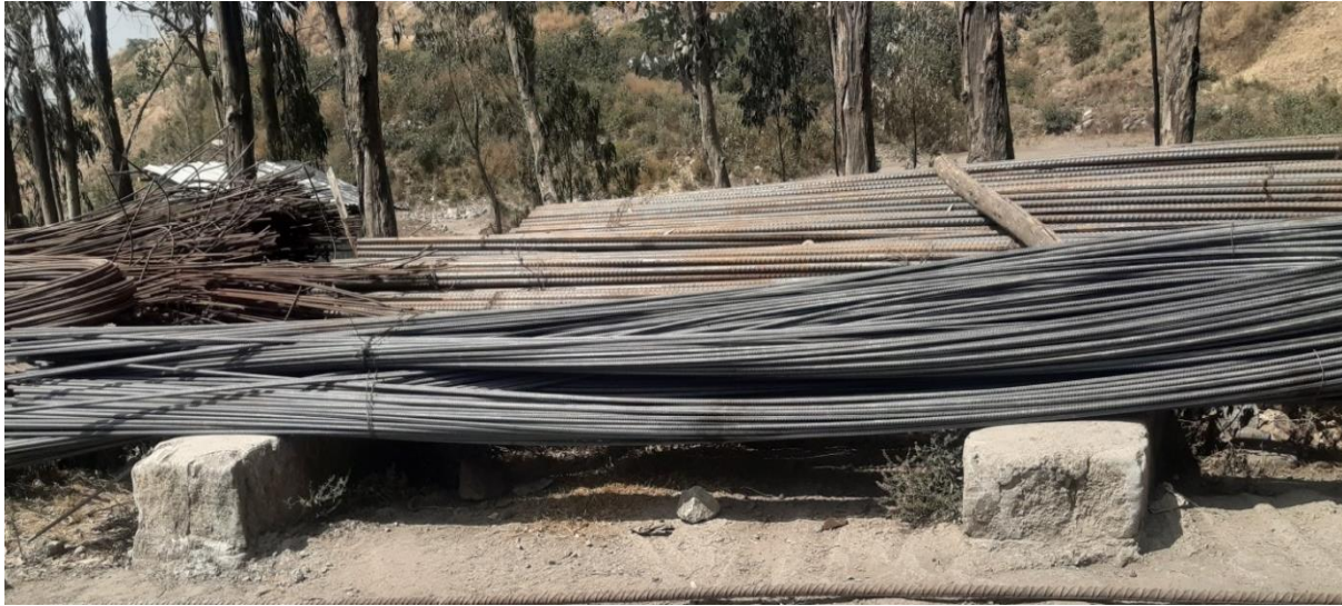
Figure 17: Rebar storage on masonry
