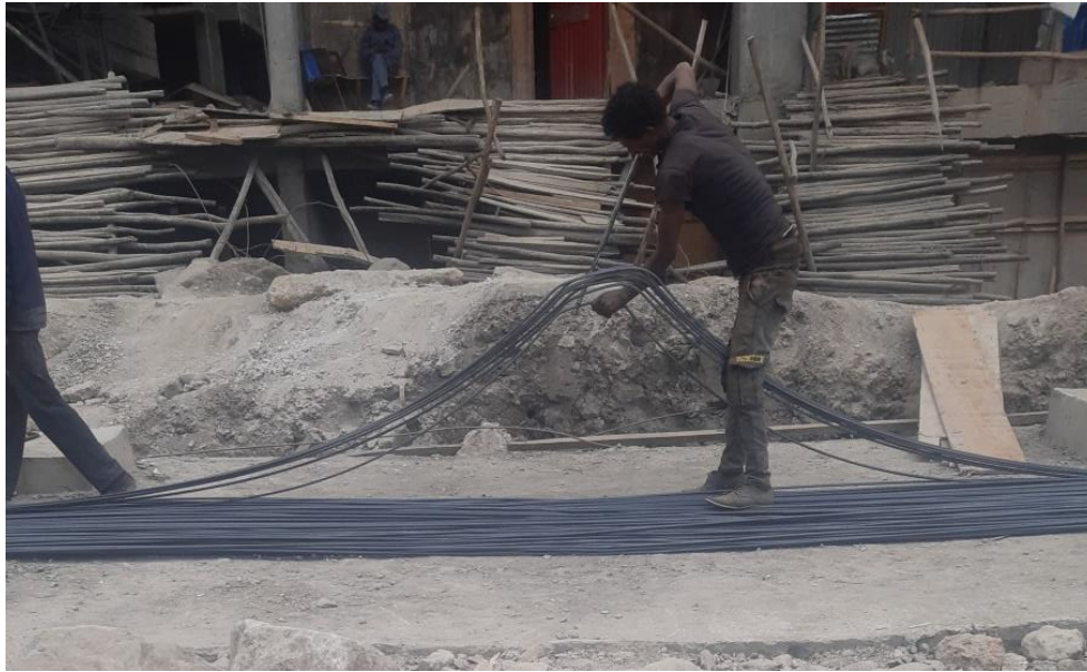
Figure 14: Rebar Straightening
