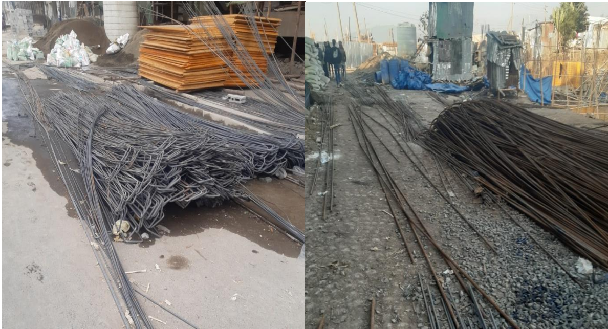
Rebar stored on the roadside
