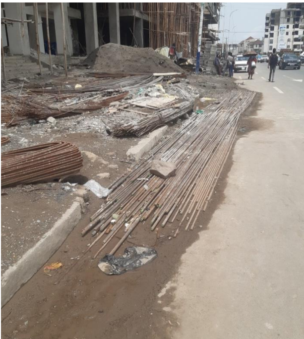
Rebar stored on the roadside
