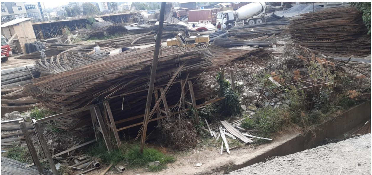
Figure 15: rebar inventory on the site
