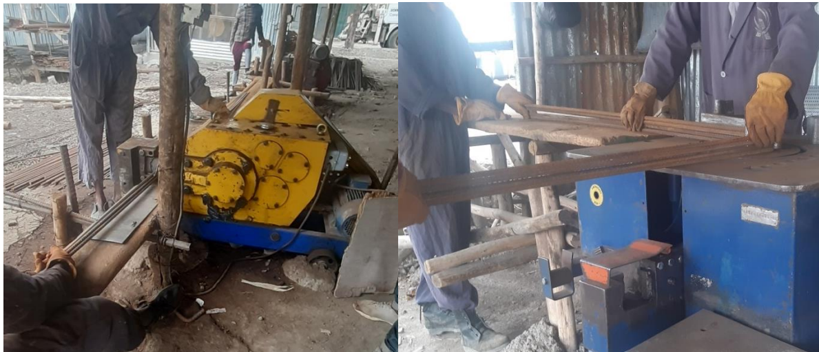
Figure 19: Off-site rebar cutting and bending
