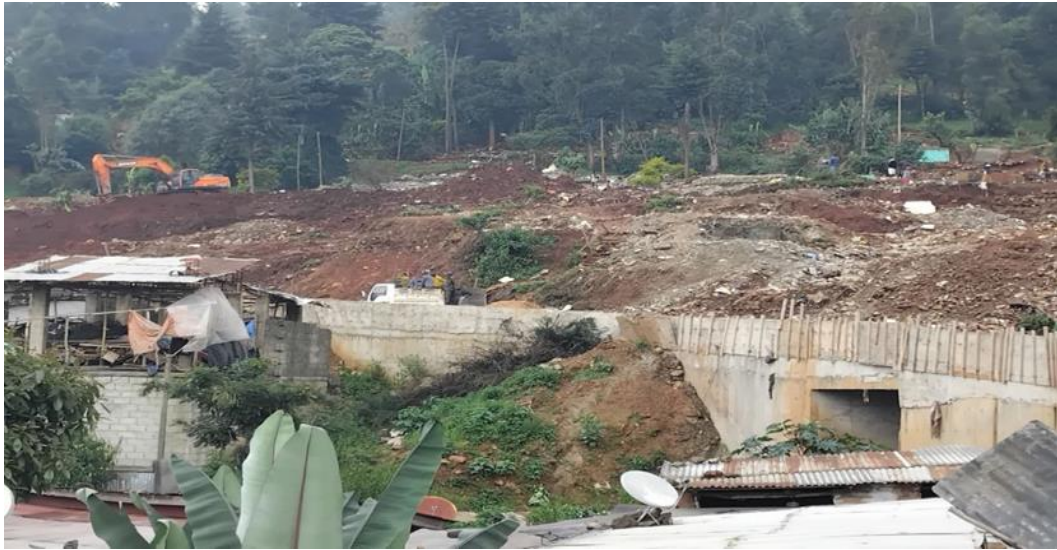
Figure 2: Yeka sub-city: demolished area after eviction have been carried out
