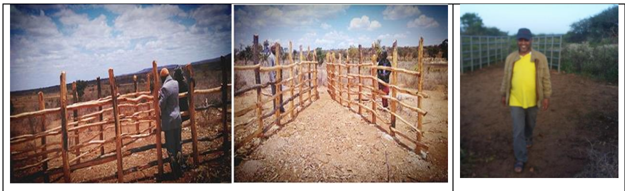
Cattle crush constructed in Masajit with local materials (Left and center) and Recent construction of crush at Haysuftu, with metal (right)
