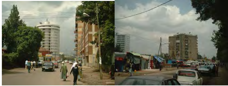
FIG. 9.6 RANGE OF BUILDING HEIGHTS IN BHERAWI THEATER AREA Source: Field Work (2005)
