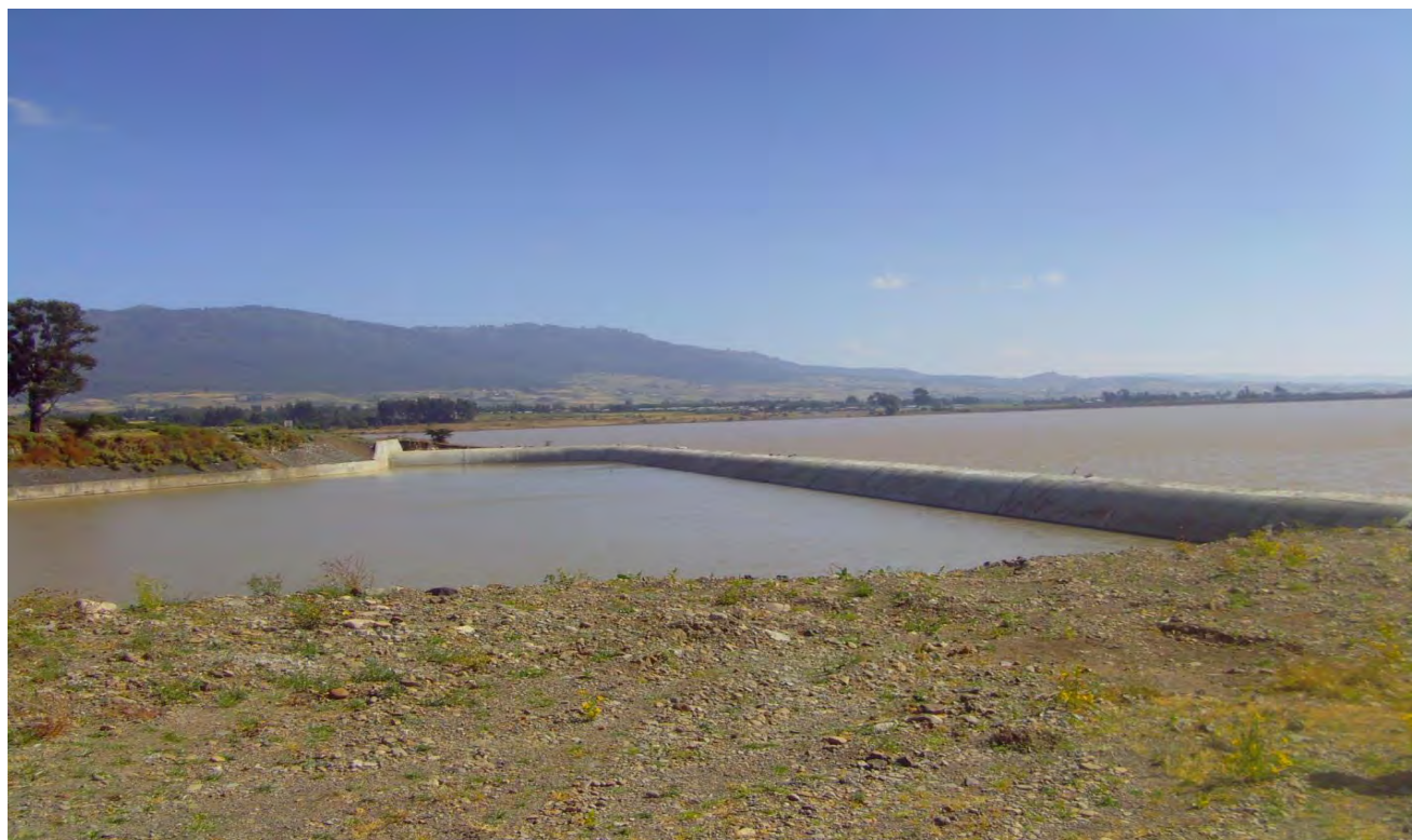
Newly constructed spillway (2.5m height from the crest of the existing spillway)
