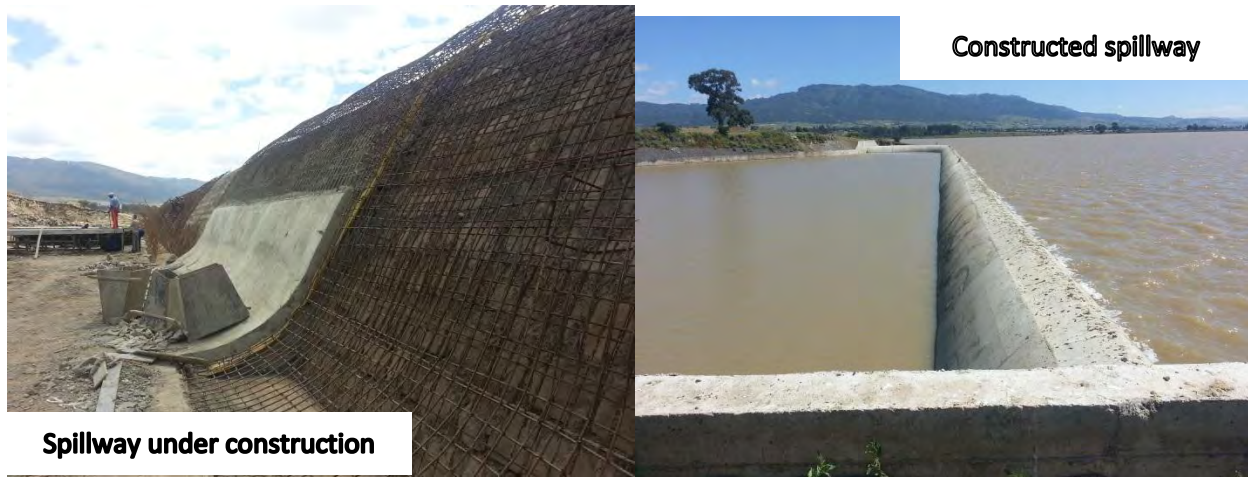
Figure 2-1: Spillway under & after construction
