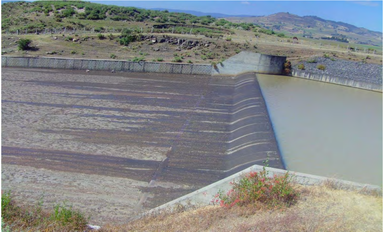
Existing spillway about 200m downstream of the new spillway
