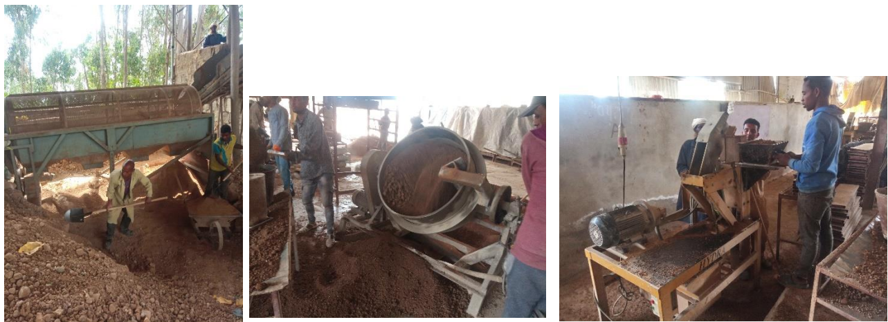
Figure 4. 17: The process of sieving, mixing and machine compression of hydraform
