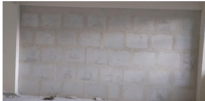
Figure 4. 15: Gypsum block construction for office partitions
