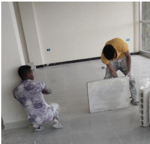
Figure 4. 15: Gypsum block construction for office partitions
