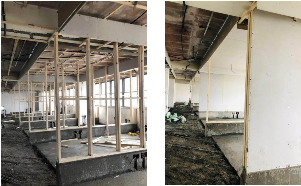
Figure 4. 19: Gypsum board construction
