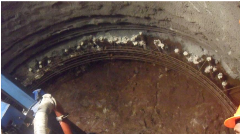
Figure 4. 3: Primary lining installation
