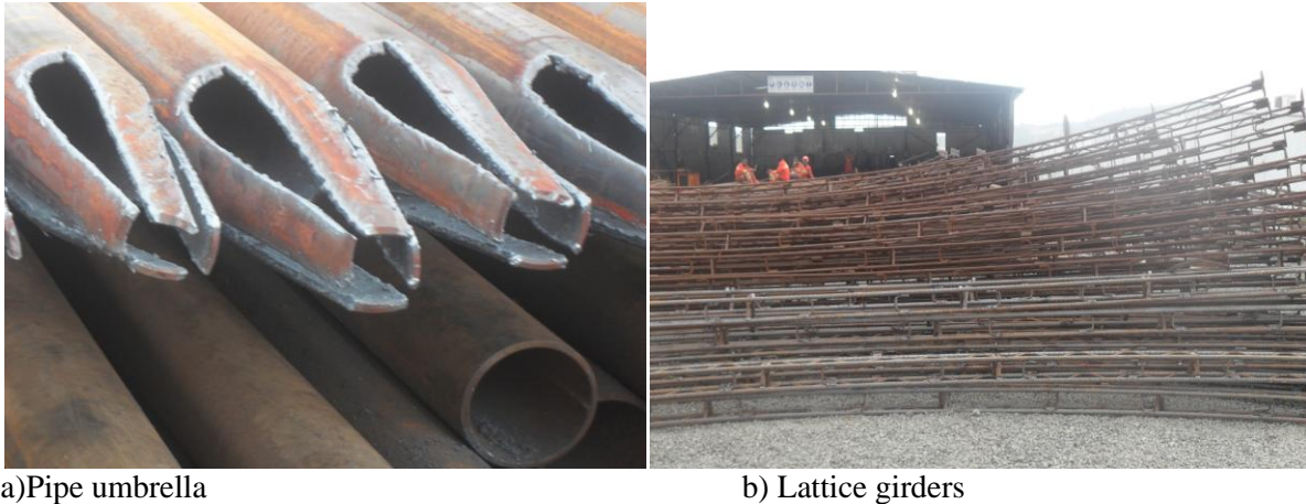
Figure 4. 2: Pipe umbrella and lattice girder used on site
