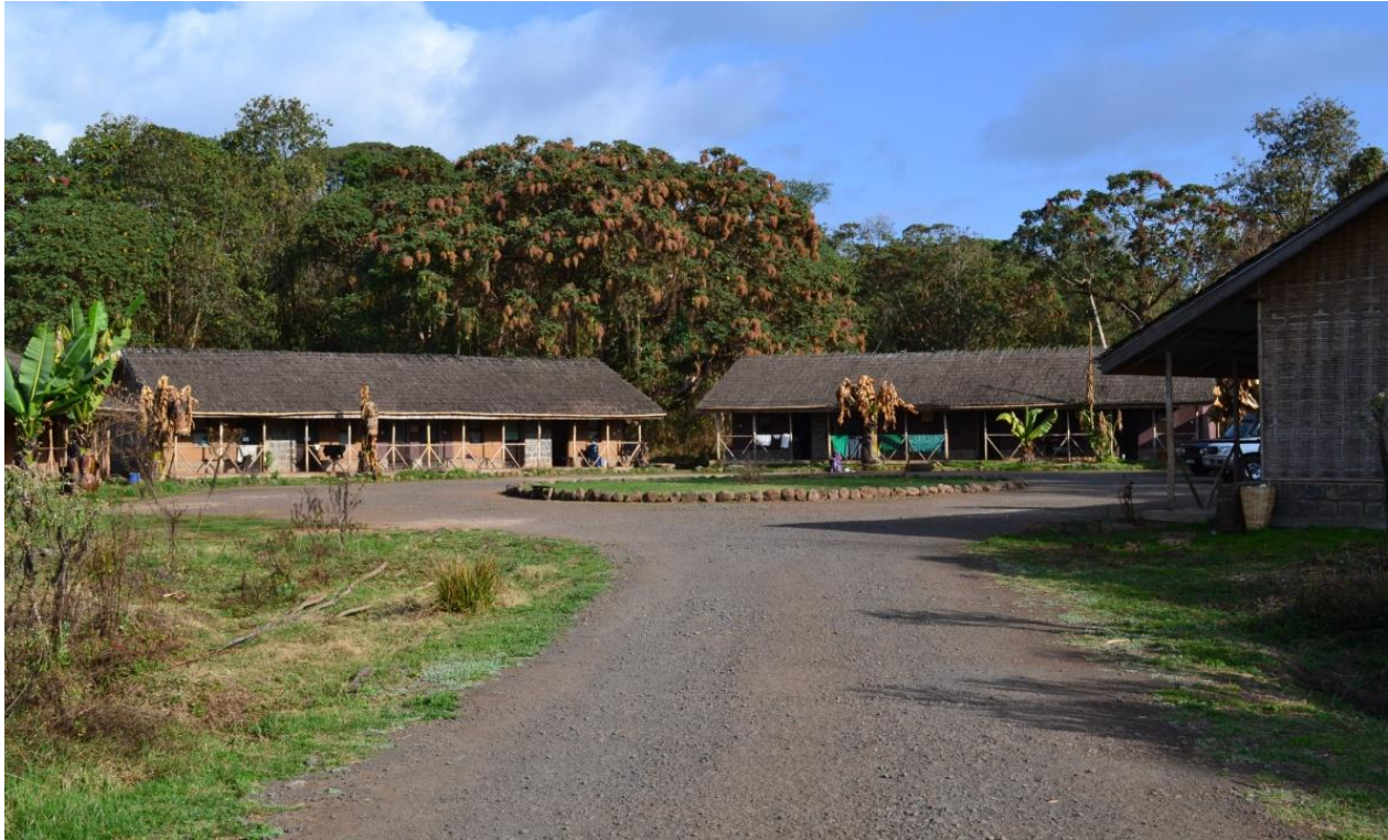
Figure 8 : Staff Accommodation at the site
