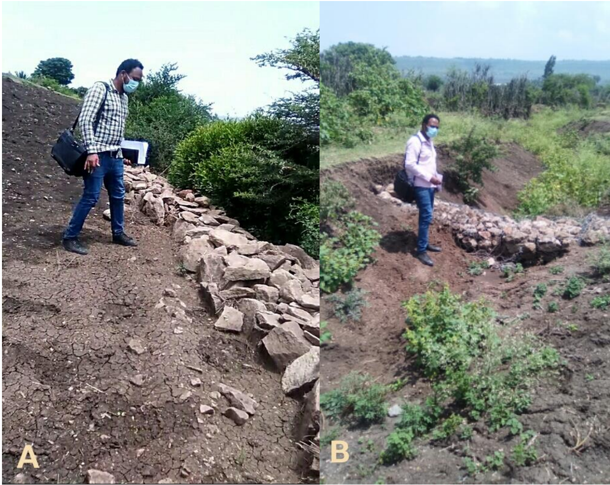
Figure 13: Photos of stone terracing on farmlands (A) and gabion check dam on gully (B)
