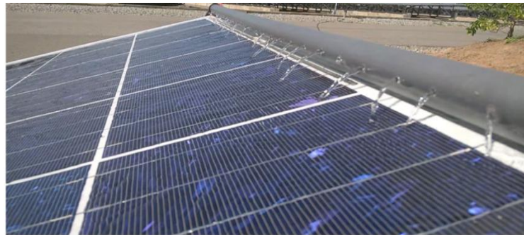
Fig.2.19. PV arrays cooling and cleaning technique (Chandrasiri, et al 2017)
