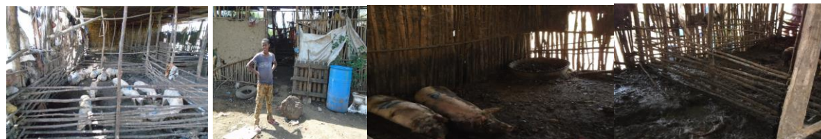
Figure 20. Poorly constructed swine barns (Photo: Kassa, 2016)
