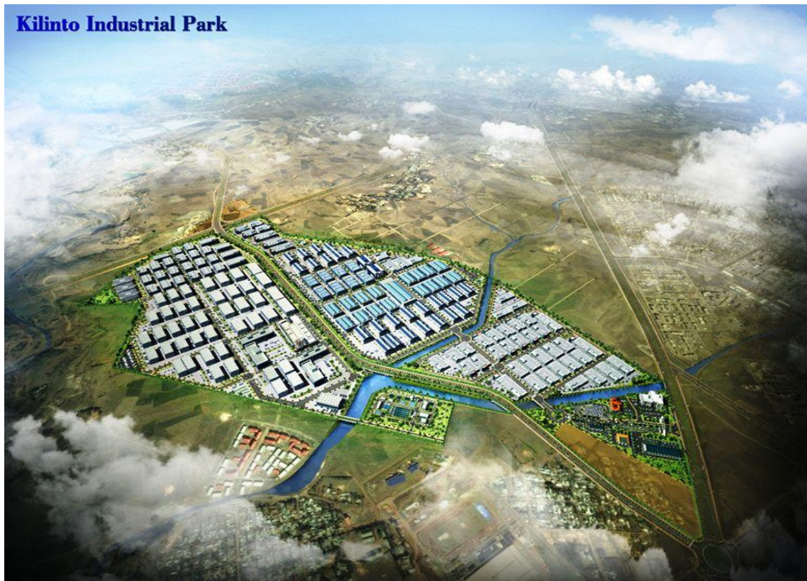
Figure 15: Kilinto Industrial Park
