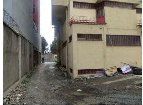
Figure 5-6 Side access to Apartment/back yard
