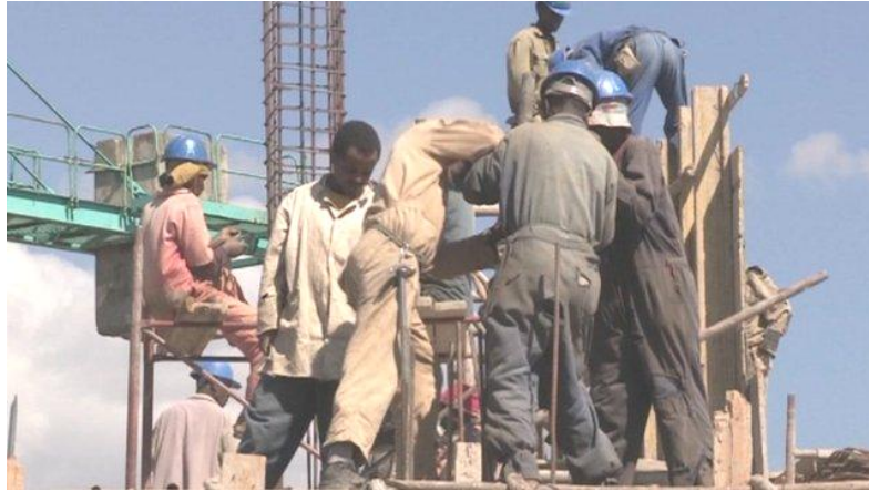
Figure 3.21 People working at construction site
