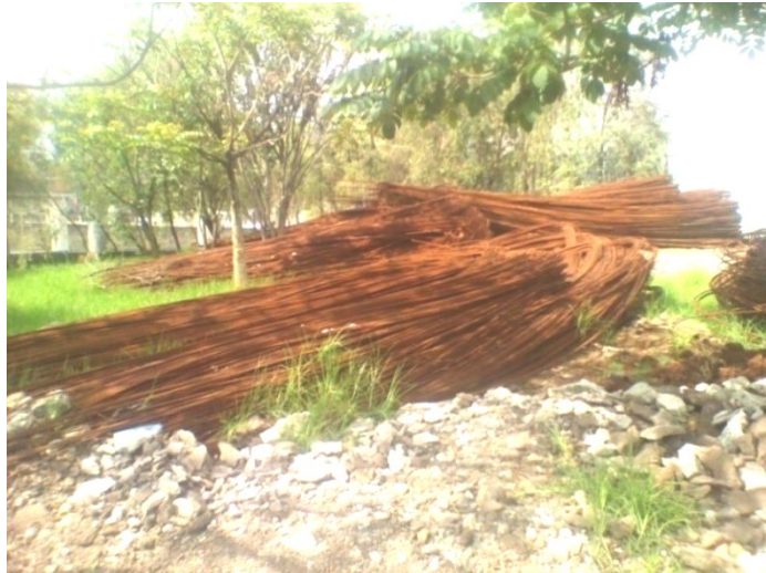
Figure 3.8 Photograph illustrating storage of reinforcement bar for construction of G+3 parking Kazanchis area, Addis Ababa - 3
