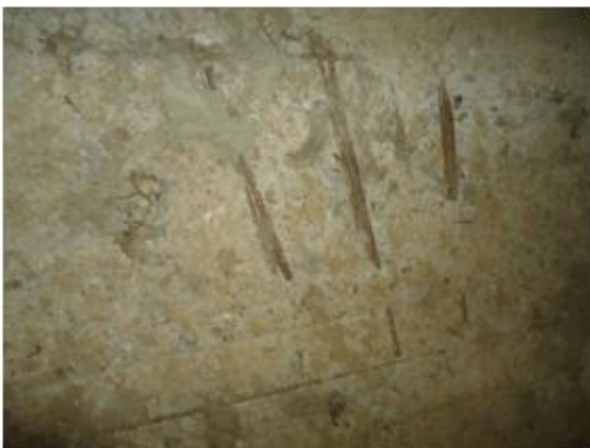
Figure 3.30 Cover concrete peel off and rebar exposure on deck slab
