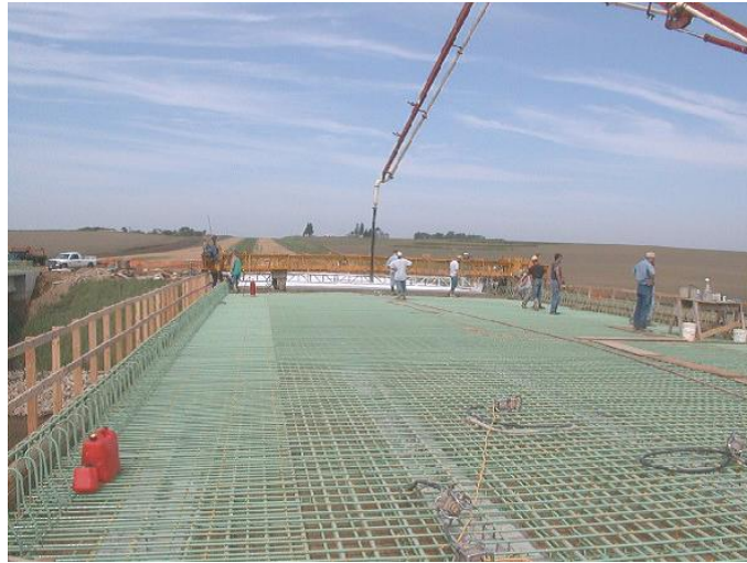
Figure 5.1 Bridge deck concrete placements (epoxy coated reinforcement bars)
