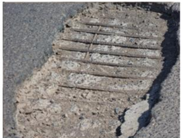
Figure 3.24 Crack and rebar exposure
