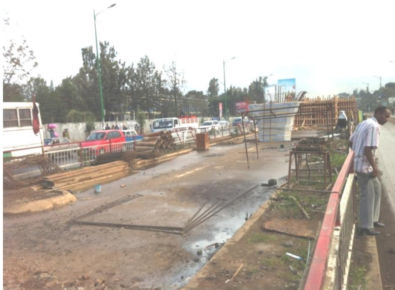
Figure 3.5 Photograph that illustrates railway project around Meskel square, Addis Ababa
