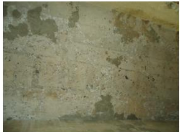
Figure 3.30 Cover concrete peel off and rebar exposure on deck slab
