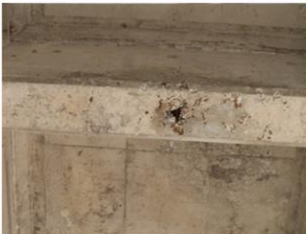
Figure 3.24 Crack and rebar exposure
