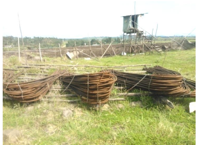
Figure 3.11 Photograph that shows storage of reinforcement bar for construction of G+6 office building around Yerer, Addis Ababa – 2
