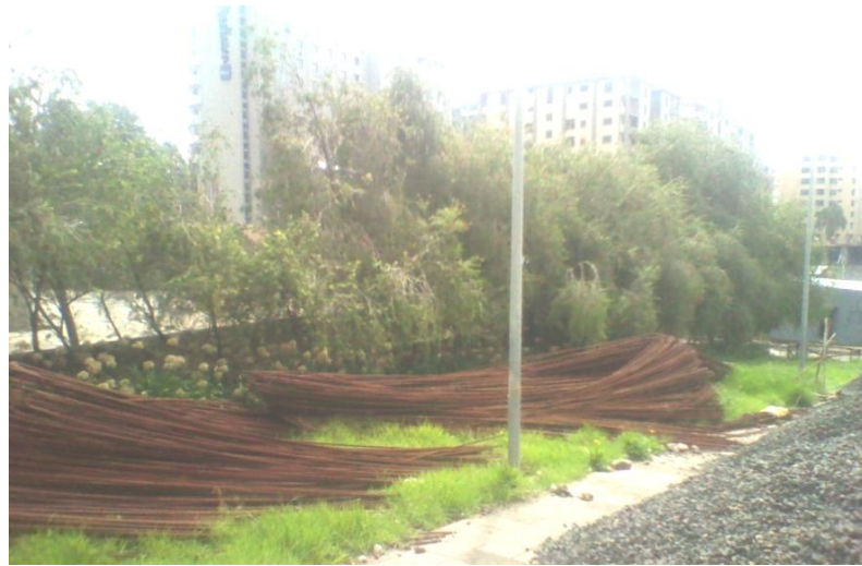
Figure 3.6 Photograph showing storage of reinforcement bar for construction of G+3 parking Kazanchis area, Addis Ababa - 1
