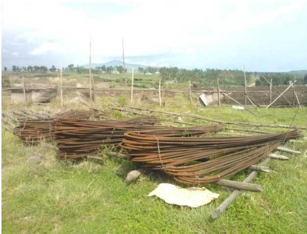
Figure 3.11 Photograph that shows storage of reinforcement bar for construction of G+6 office building around Yerer, Addis Ababa – 2
