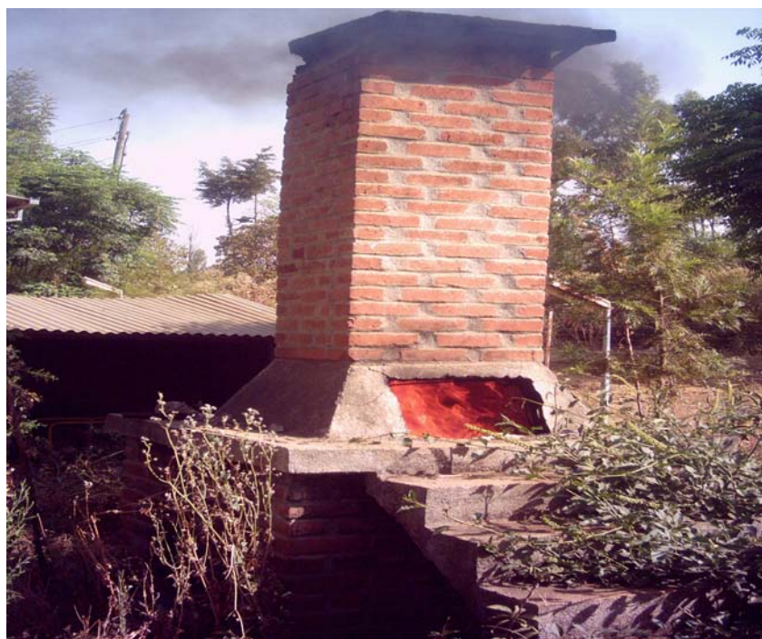
Fig 4 .HCW burning with incinerator in Durebetie health center
