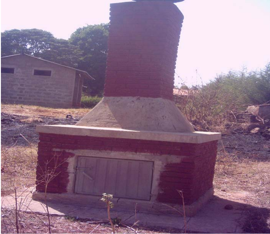
Fig 5. Newly constructed incinerator for HCW disposal in Dangila health center
