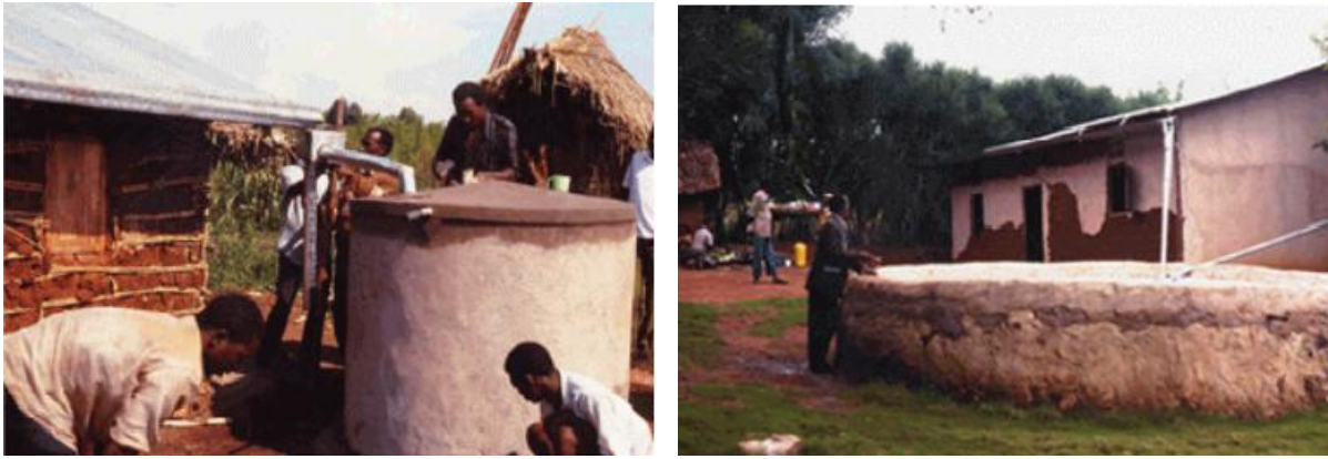
Figure 3- 4 : (a) (b) Rainwater tanks constructed by local builders
