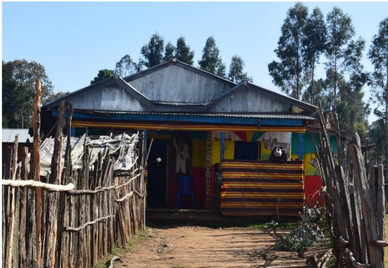
Figure 4-2: Building condition analysis, Photograph by author, March 2020.
