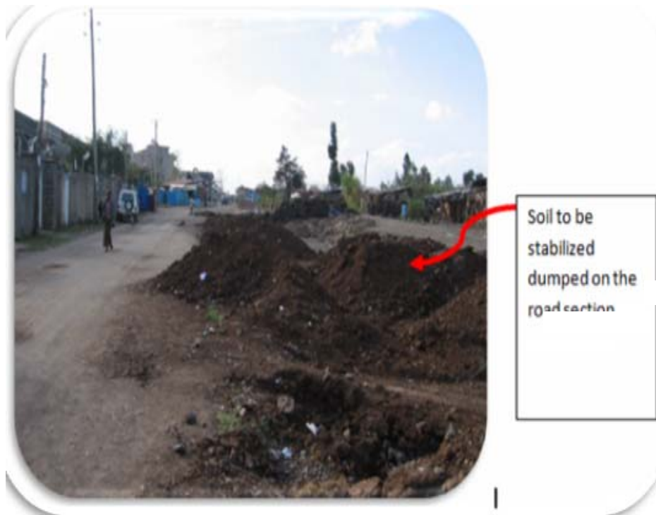
Figure 4.10: Soil transported to the road section for grade adjustment & stabilization (Around Bole High School)
