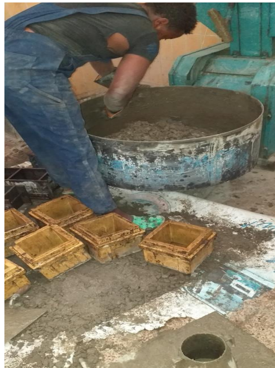
Photo 12. Concrete ingredients being mixed.
