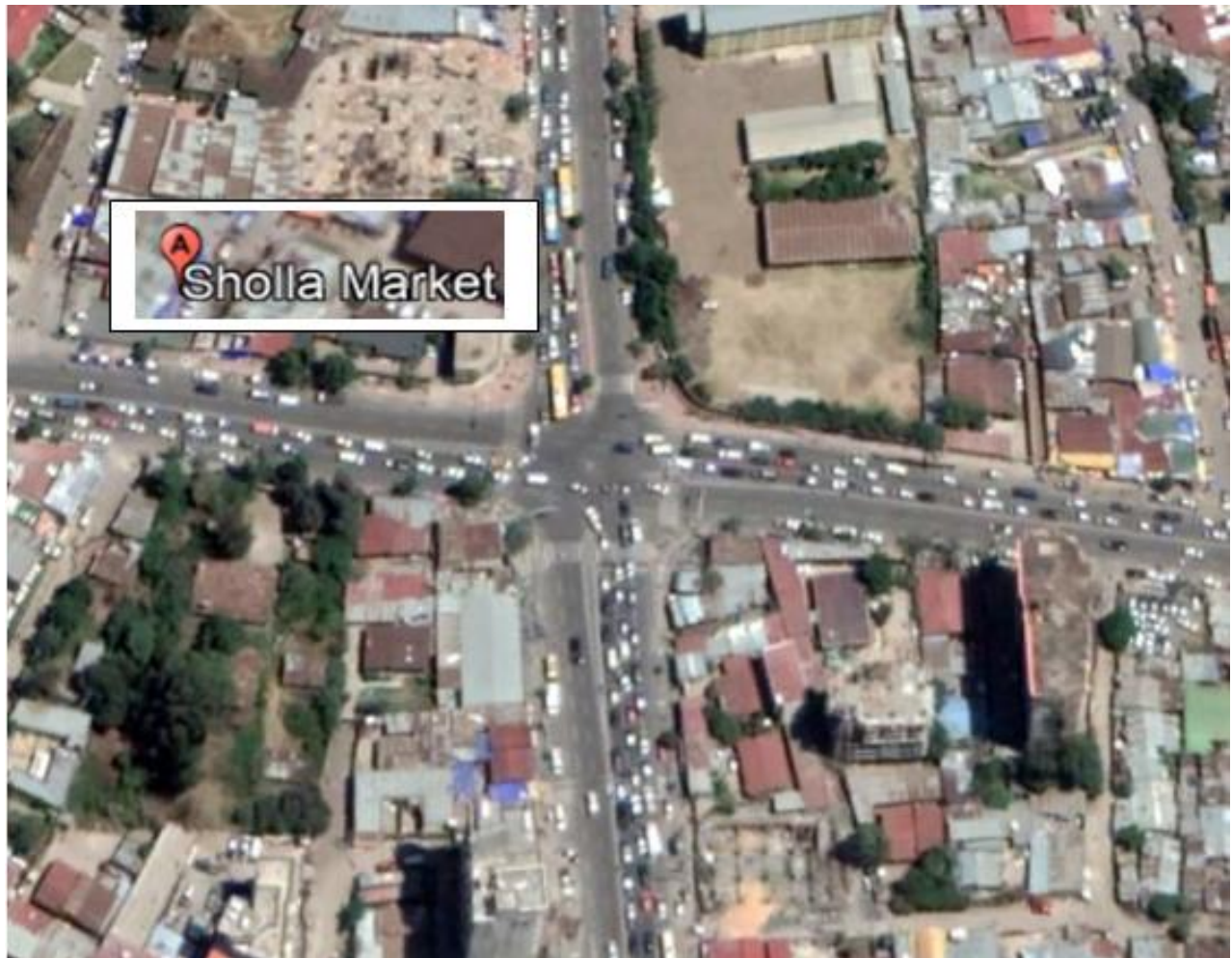
Figure 3. 5 Aerial photo of Shola Signalized Intersection
