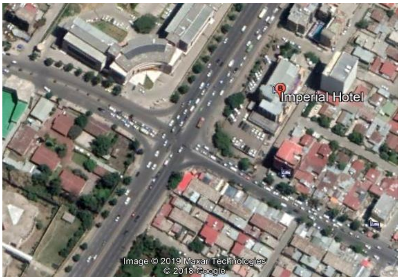
Figure 3. 6 Aerial photo of Imperial Signalized Intersection
