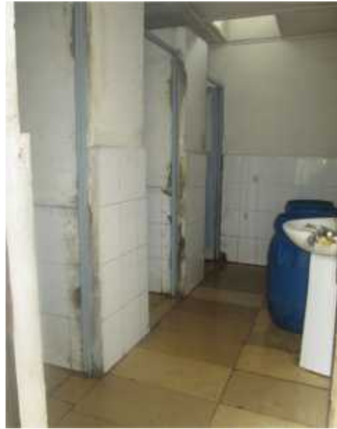
Figure 4.10: inside the toilet and inaccessible stall
