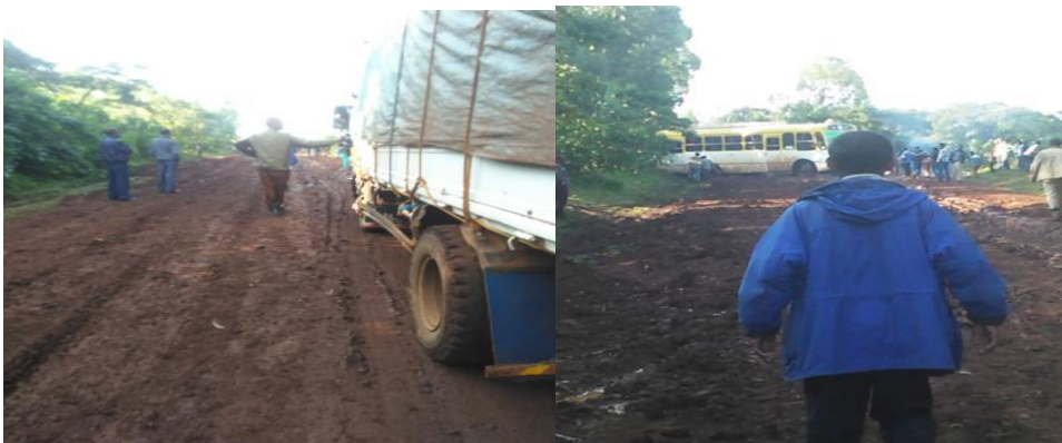
Figure 4.2: Road damage and its effect on public transportation
