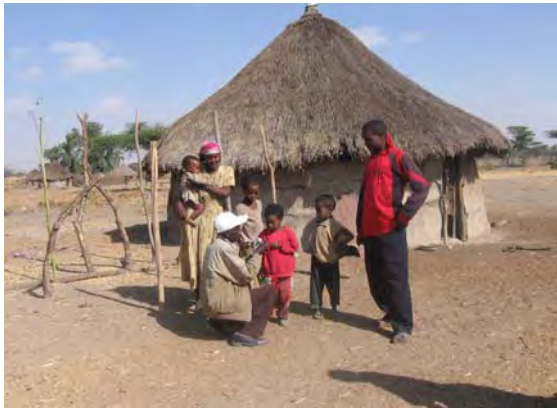
A) Grass top and mud wall reinforced with wood.
