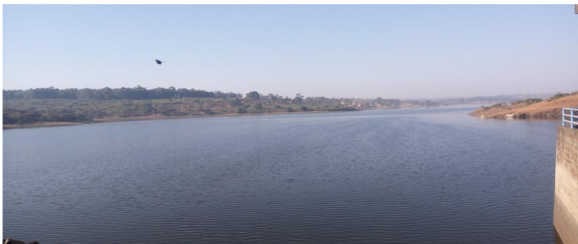
Figure 2:2 Finchaha Hydro Power Plants dam
