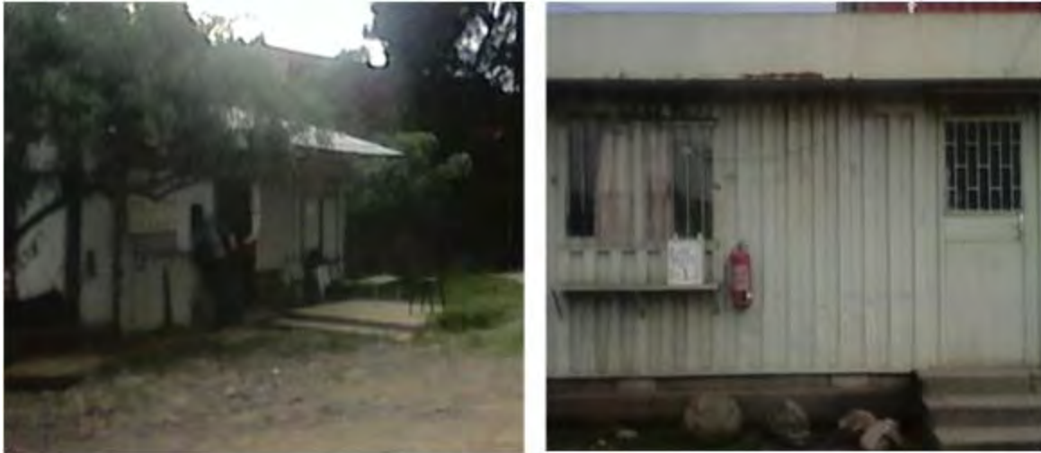
Figure 4. Office facilities for dry port employees
