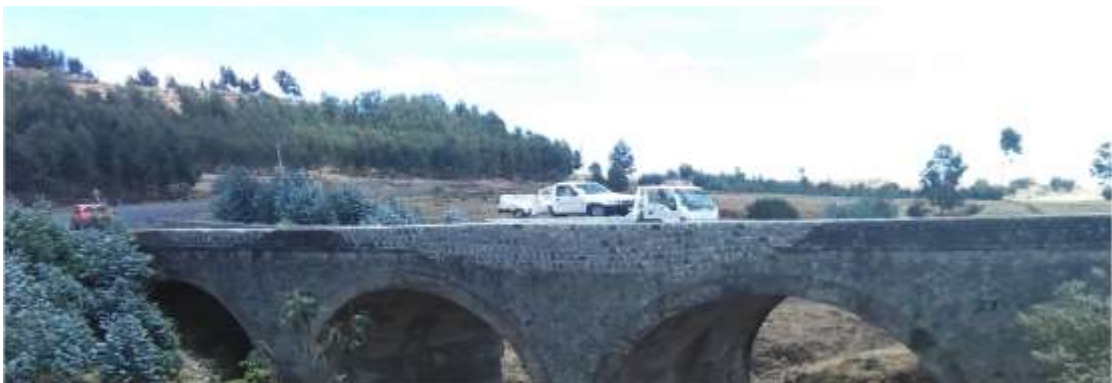
Figure-14: Sostaf Dildiy near Aleltu (an arch bridge with three boxes).
