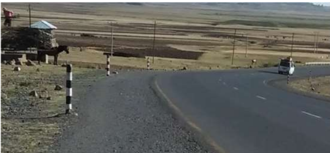
Figure-25: Chefanen road feature showing the ingress of carts at speed road.
