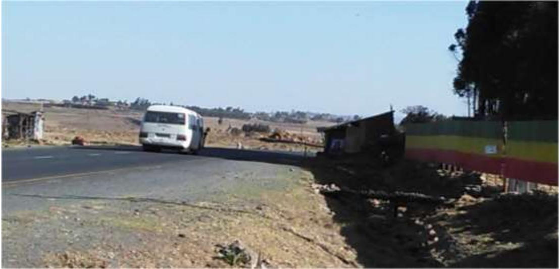
Figure-23: Chefanen road feature around the church and sight distance with low visibility problem
