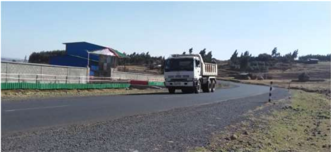
Figure-24: Chefanen road feature around beer (local Areki) factory.
