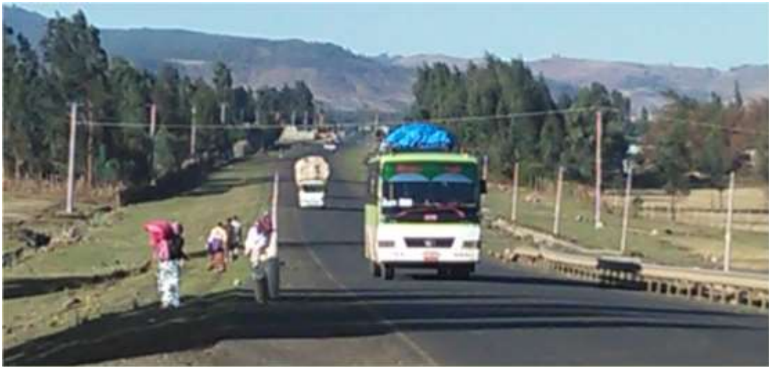
Figure-18: Flow of vehicles at Dabie and the long tangent with no walkways.
