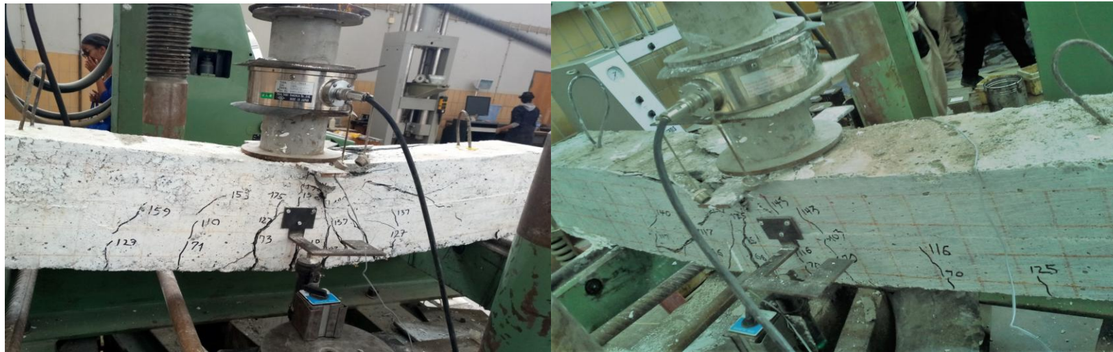
Figure 4-5 Flexural failure and crack pattern observed for SCB3(left) and VCB3(right)
