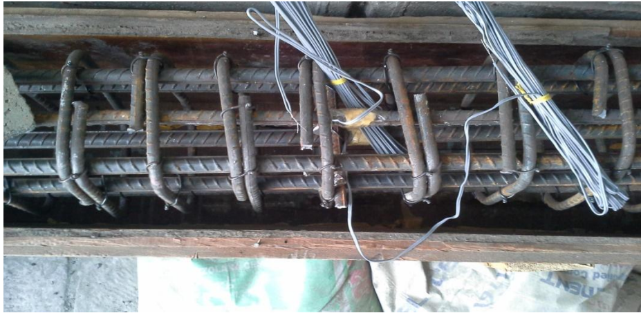
Figure 3-5 Specimen preparation, formwork, and steel reinforcement
