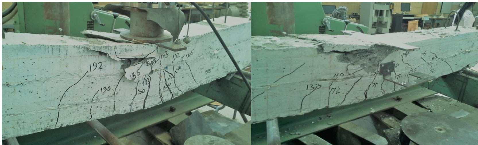
Figure 4-3 Flexural failure and crack pattern observed for SCB2(left) and VCB2(right)
