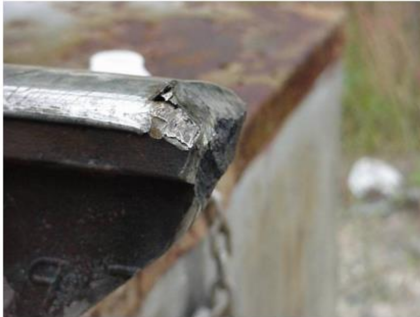
Impact Batter from Rolling Stock Wheels
