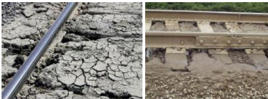
Figure 2-11 Ballast Fouling [30].
