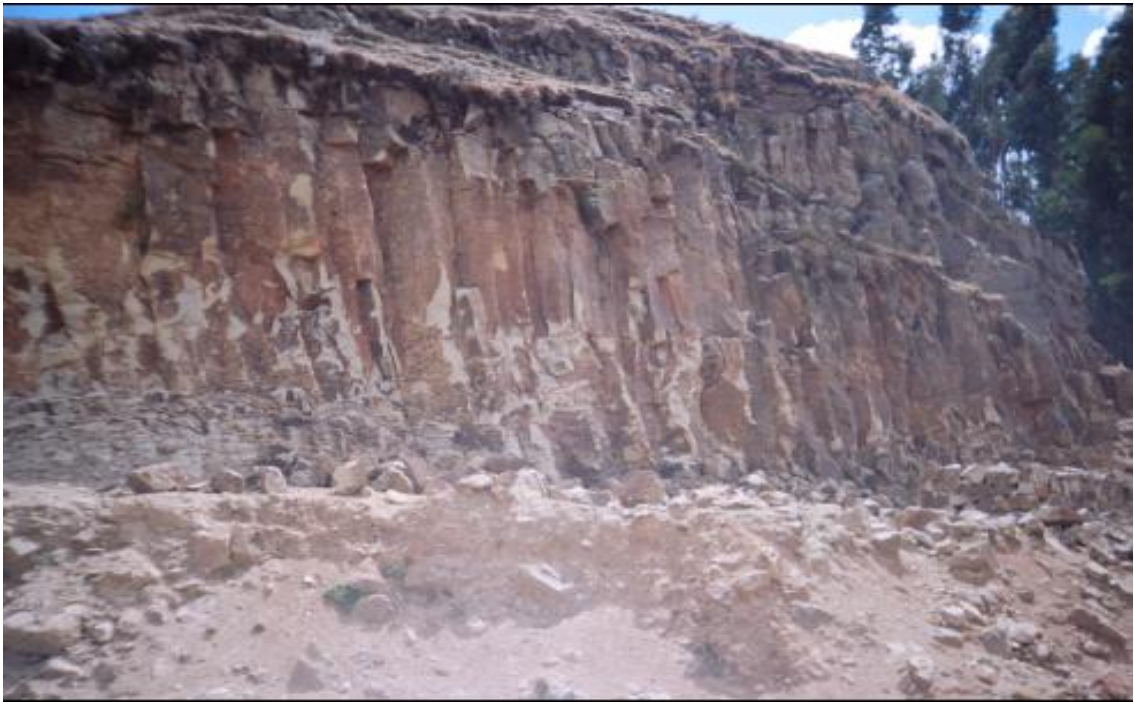
Plate 4. 2 Weathered, fractured and jointed Rhyolitic ignimbrite at Keba area
