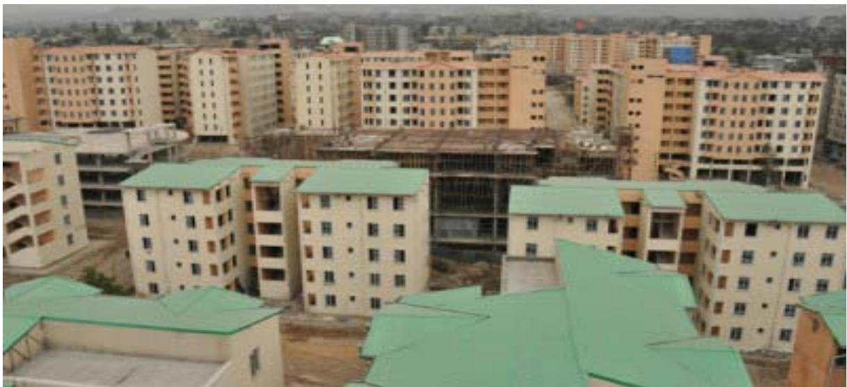
Figure 2: Bole Bulbula condominium site
