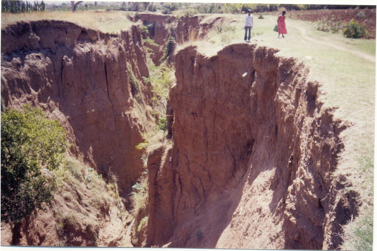
Figure 8. One of the Recent Cracks in Muleti area.
