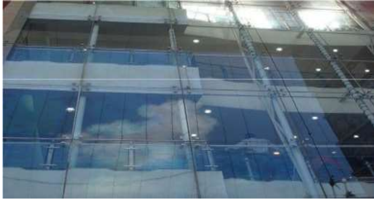
Figure (b). Truss supported PFGFS covering a 4-storey building
