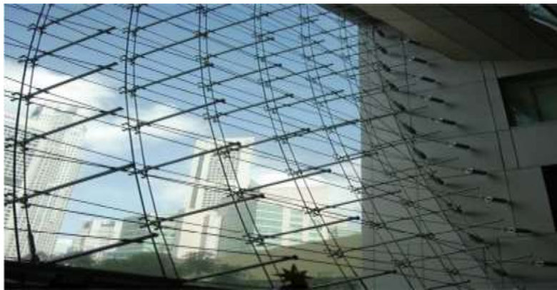
Figure (c). Cable supported PFGFS
