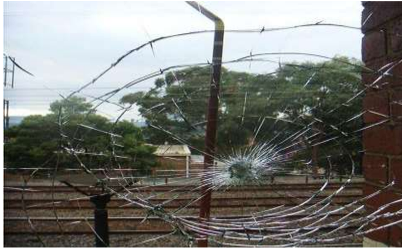
Figure 2.3: Crack pattern of heat strengthened glass (source Tom castle, 2012)
