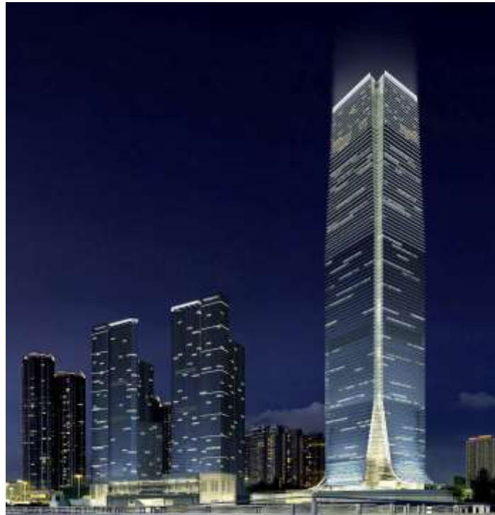
Figure 1.4: 290m height, International Commerce Centre, Hong Kong, China (Right hand side), which will be the tallest building in Hong Kong.
