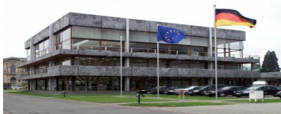
Figure 2- Exterior view: Constitutional Court of Germany. 72
