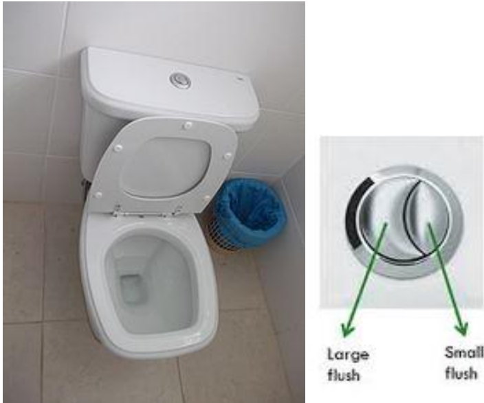
Picture 3) Dual or double flush toilet
