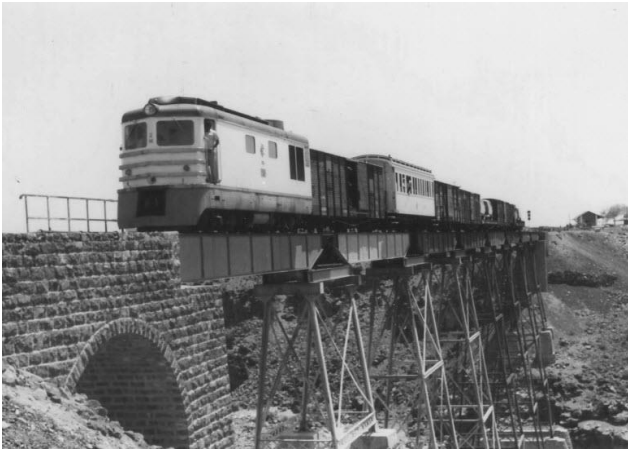
Figure 1: Ethio-Djibouti Railway Diesel locomotive with a mixed goods/passenger train on the Holhol viaduct in 1960[1]
