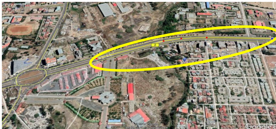
Figure 6: Segment 1 (Sealite Mihiret Station to Civil Service station), 0.77 KM
