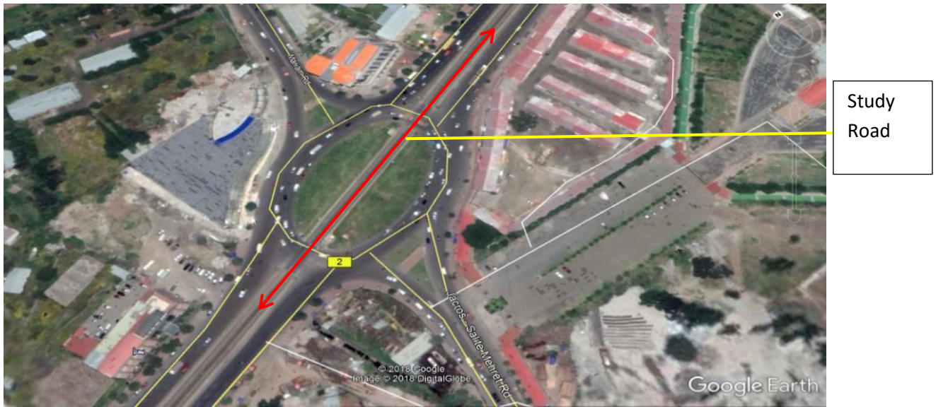
Figure 4: Sealite Mihiret Roundabout
