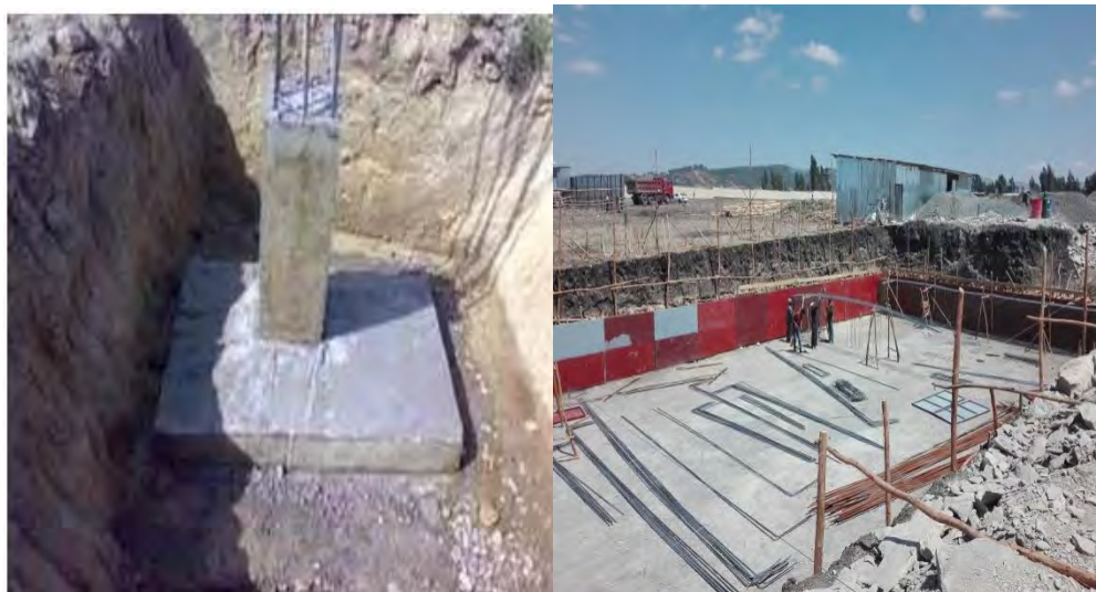
Plate 3.1 Spread (Isolated) Footing Plate 3.2 Mat Foundation
