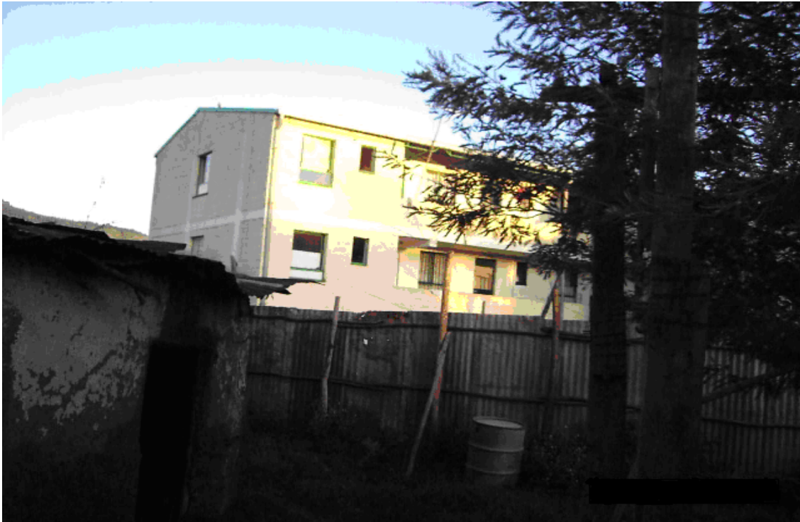
Plate 6. Condominiums constructed in Arada sub-city locality.
