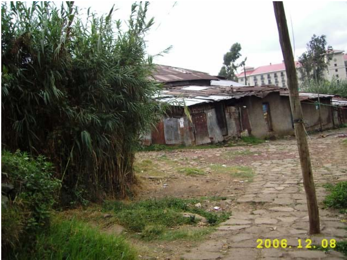
Plate 12. and 13. Poor quality and dilapidated houses around Sheraton Addis Hotel.
