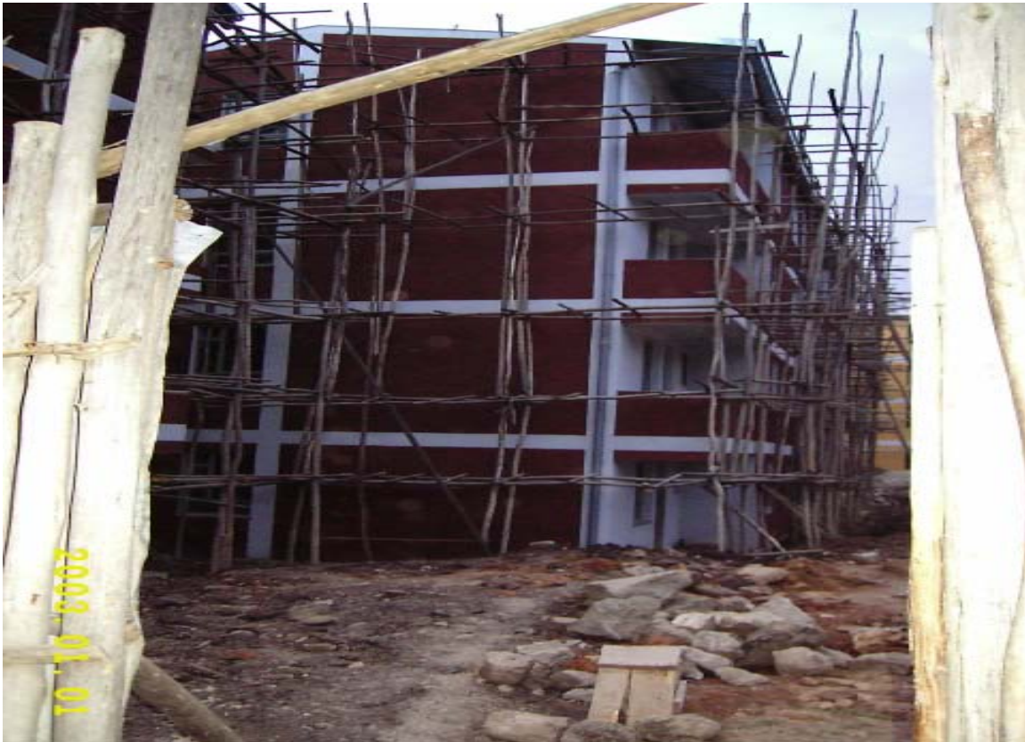
Plate 7. Condominiums under construction in Yeka sub-city.
