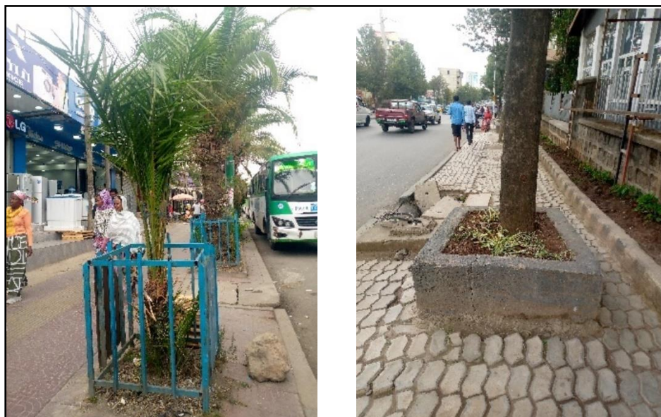
Figure 4.9 Adaptive measures taken - protective structure
