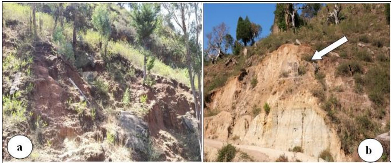
a) Translational slides showing the surface of rupture at the debris-bedrock Boundary b) Translational slide along reddish to yellowish horizontally bedded sandstone
