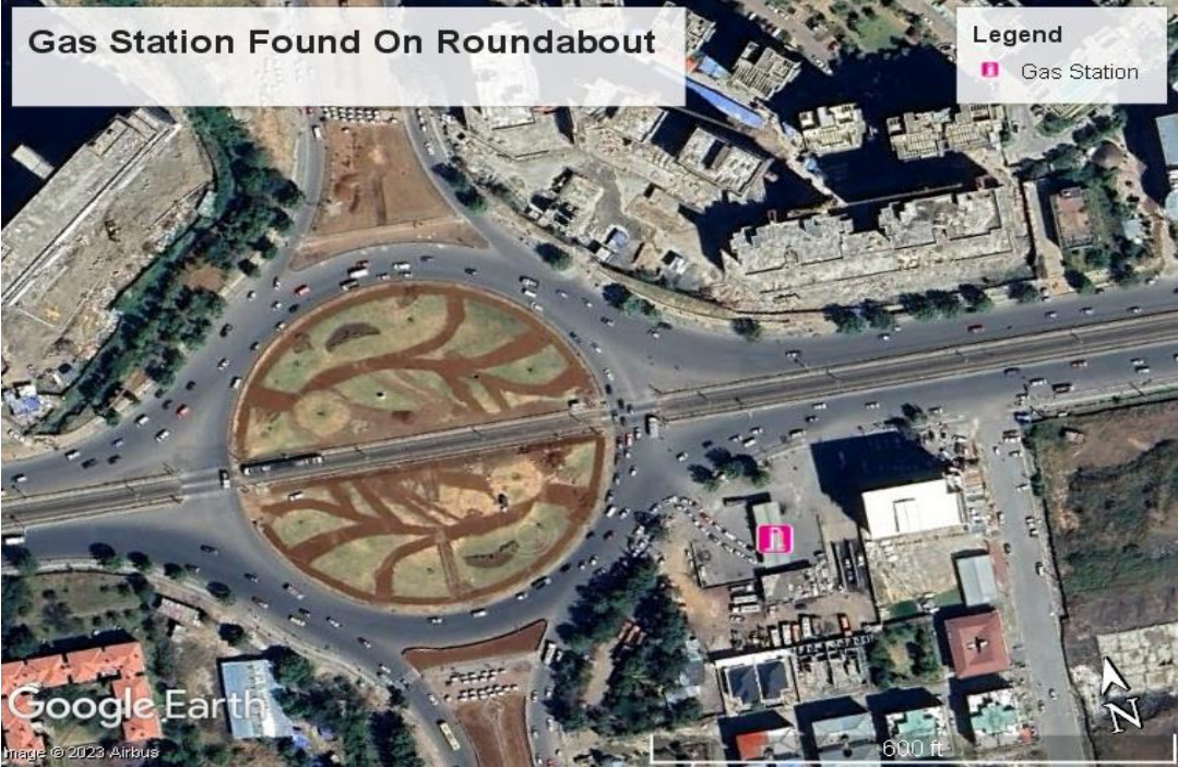
Figure 4-13 example of Fuel Station found on roundabout (Source: Google Earth (2023))
