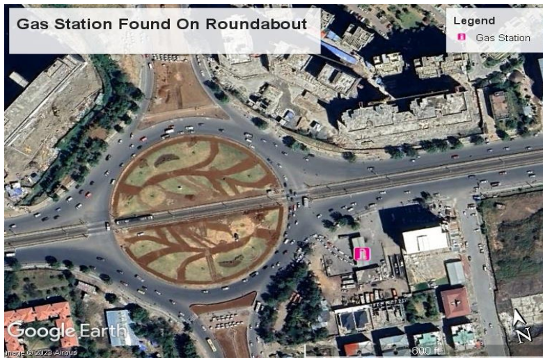
Figure 1-13 example of Fuel Station found on roundabout (Source: Google Earth (2023))
