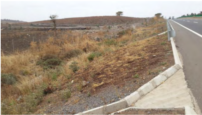
Figure2.7: Example of a fill batter road side easily blending with the surrounding landscape
