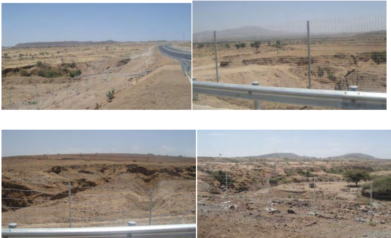
Figure 2.4a: Pictures of eroded gullies
