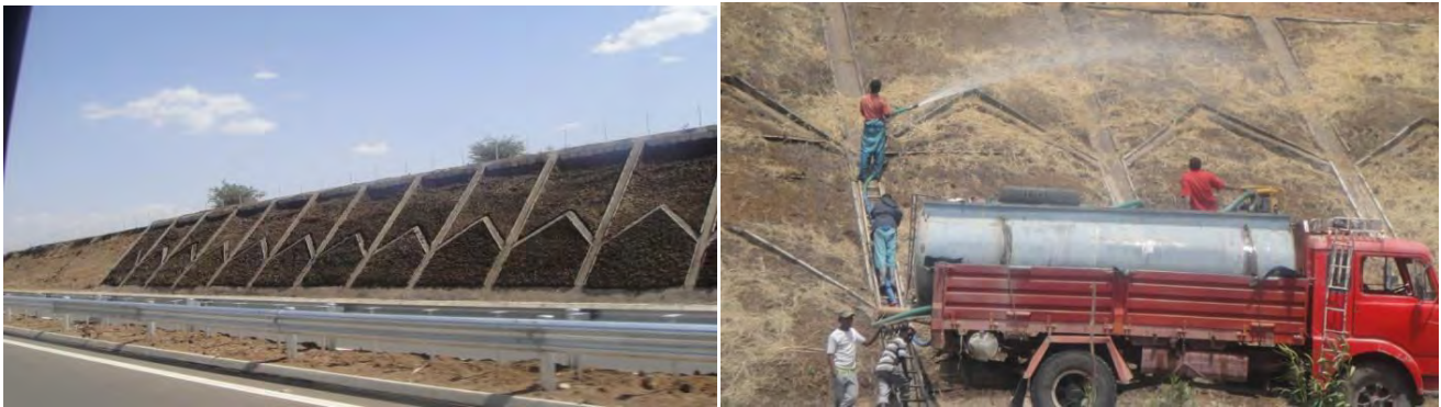
Figure 2.6: Examples of efforts to stabilize cut batters of the Express
