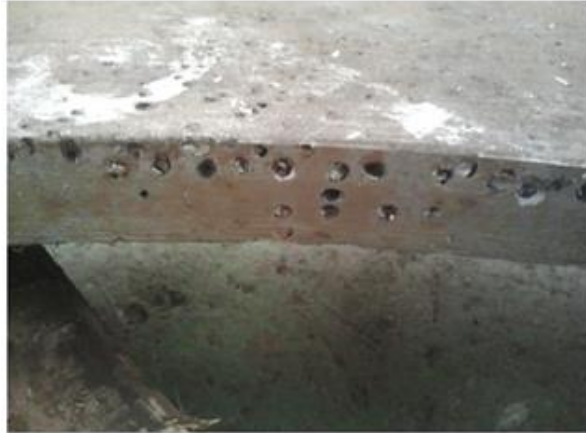
(g) Internal wall after final grinding
