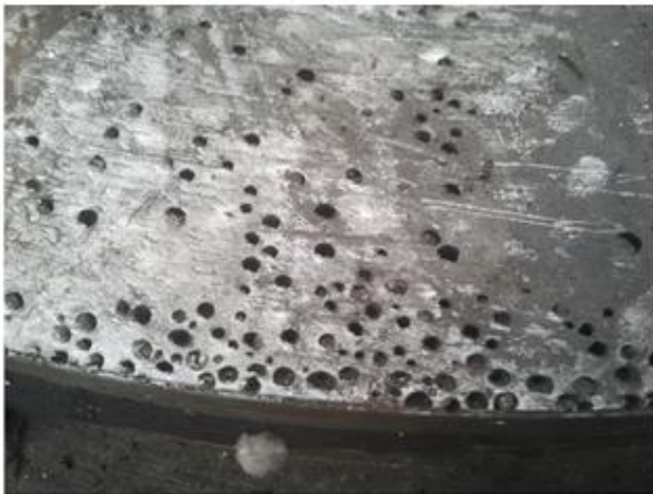
(c) Voids on the top surface
