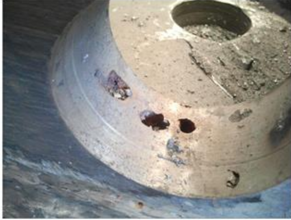
(a) Blow holes on internal surface
