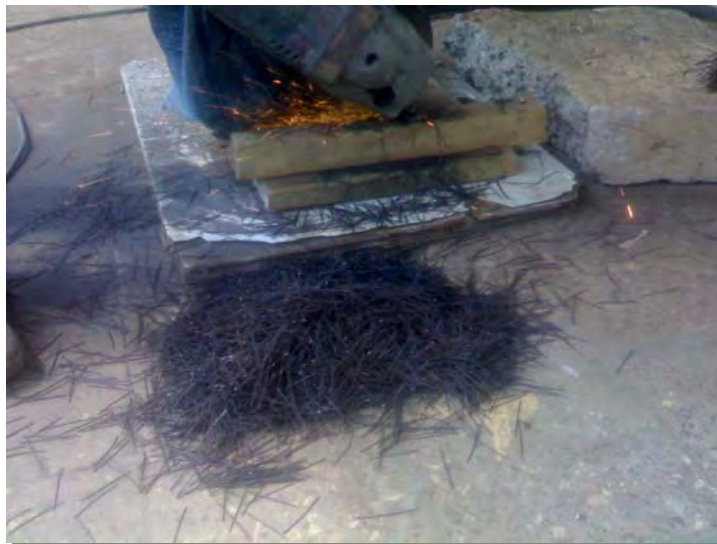
Fig. 4.2 Cutting the steel fibers to the required length.
