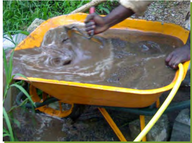
Fig. A.J-14 Washing the Fine Aggregate
