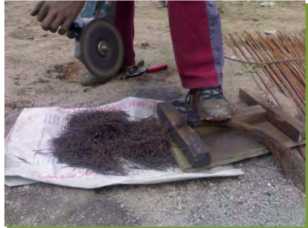
Fig. A.J-8 Cutting the Steel Fiber
