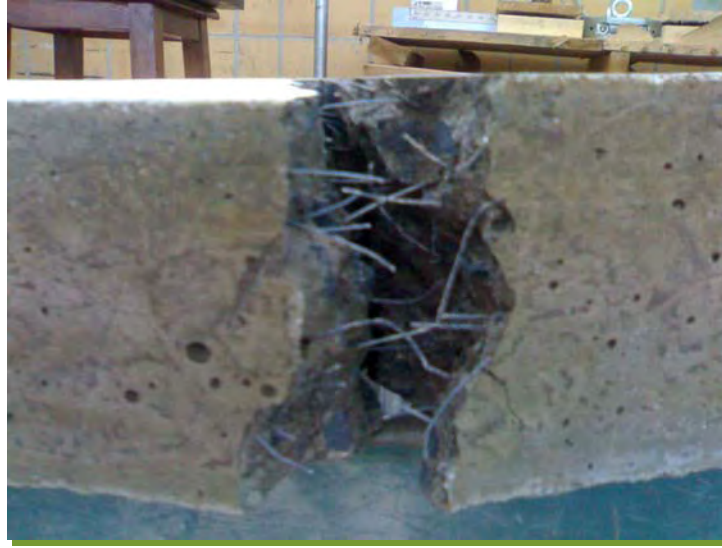
Fig. 5.10 A beam sample failed in flexure by fiber pull out
