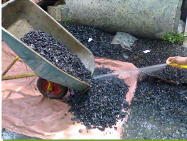
Fig. A.J-13 Washing the Coarse Aggregate
