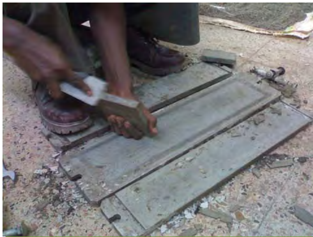
Fig. A.J-21 Cleaning Beam Mould
