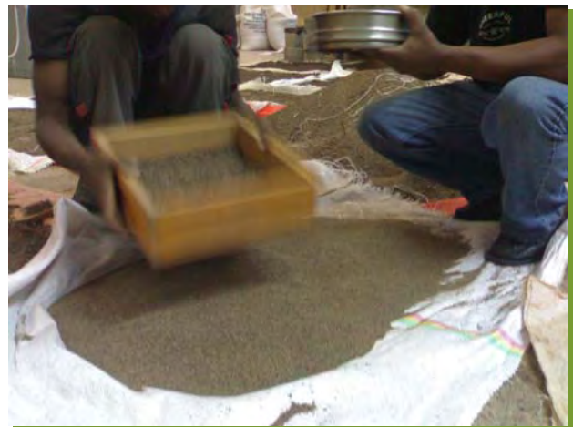
Fig. A.J-16 Sieving the Fine Aggregate
