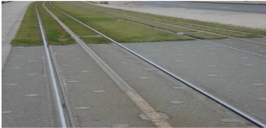
Figure 1.1 Third rails is located between the two running rails [6].
