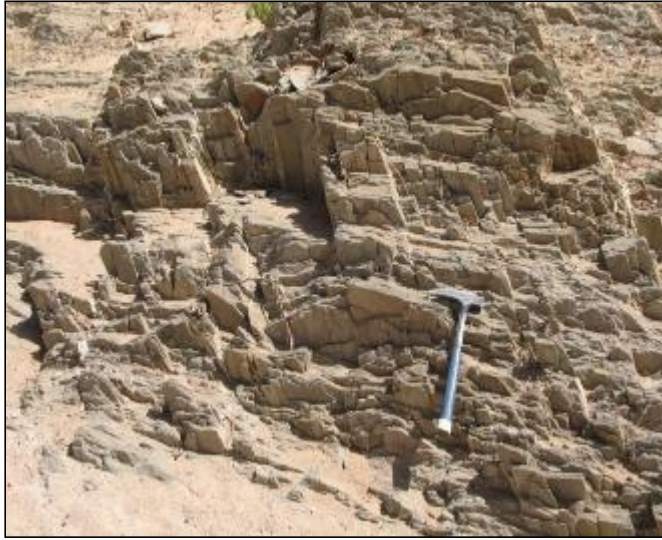
Figure 3.2: Highly fractured basement rock found to occur at the eastern foothill of Karamara mountain range
