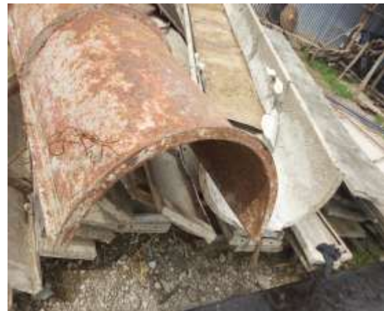
(b) Steel column panels store poorly at site
