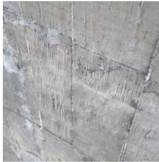
(b) Impact on surface of concrete slab
