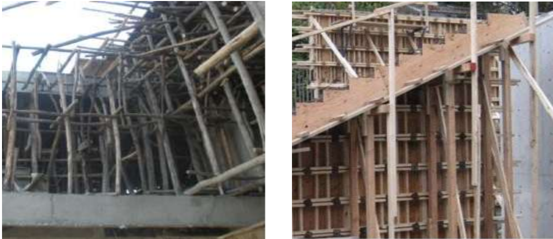
Figure 2.7 Traditional formwork constructions (Swapnali & Karke, 2016)
