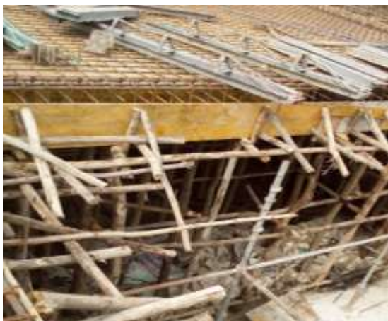
(a) Timber & steel props, plywood form
