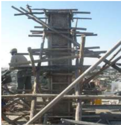
(c) Unsafe column casting
