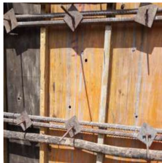
b) Using tie rods
