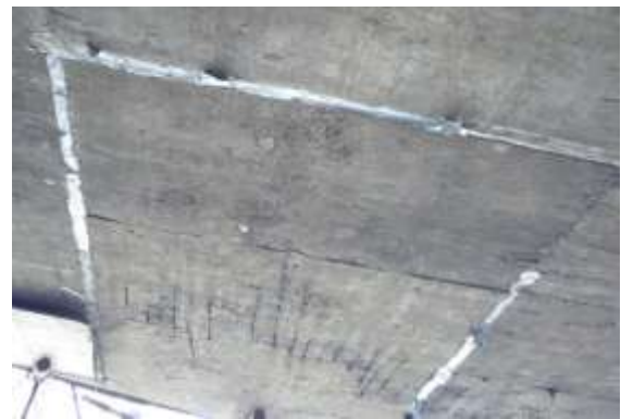
a) Poor form joint treatments and resulting concrete surface in some sites by local contractors
