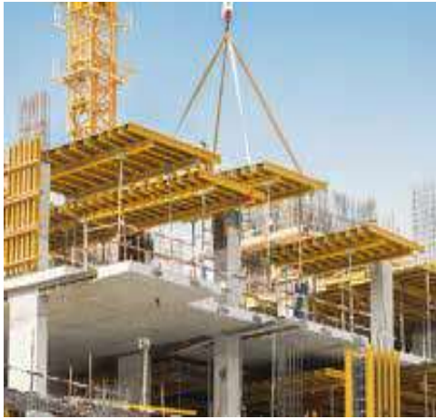
a) Assembling table form at site
