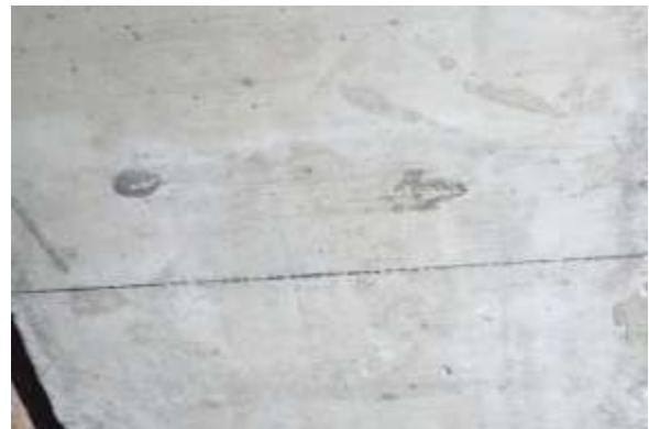
b) Tight form joints and resulting smooth concrete slab surface by international contractors
