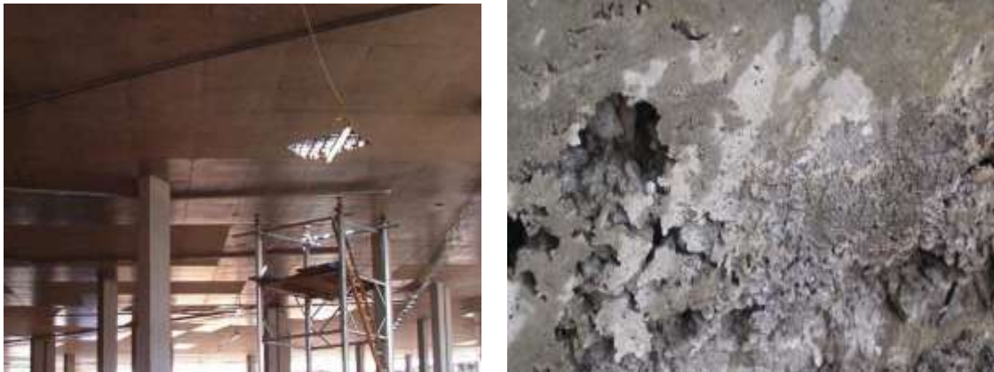
(a) Smooth and flat concrete finish
