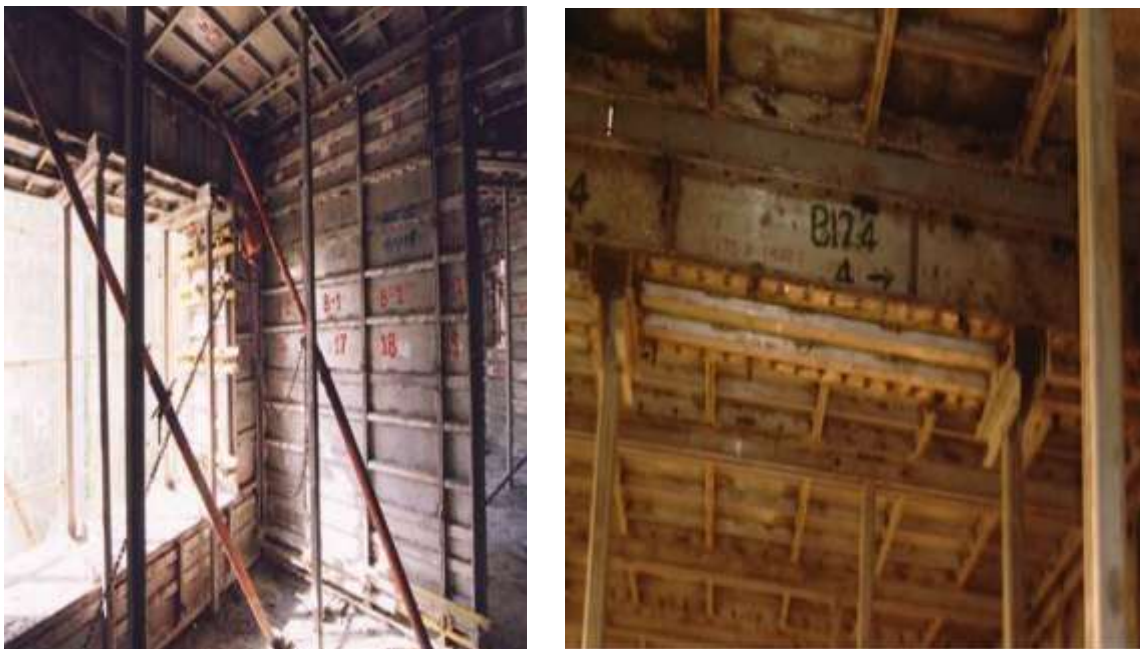
Figure 2.9 MIVAN Aluminum formwork (Swapnali & Karke, 2016)
