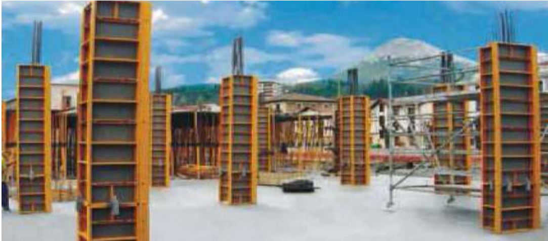
Figure 2.11 High column formwork systems (Indian ministry of rail ways, 2017)
