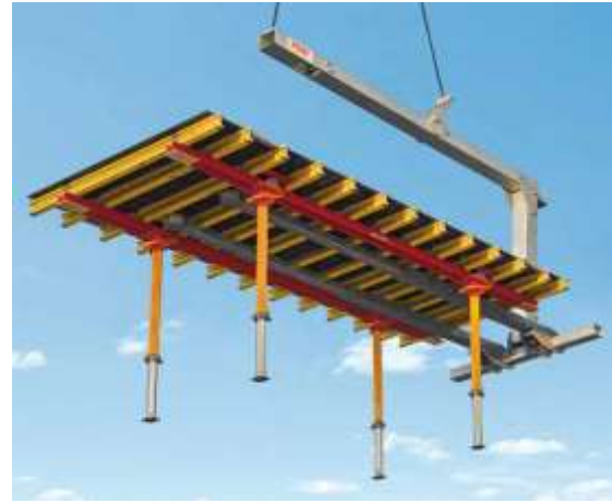
b) Moving (lifting) the table to upper storey
