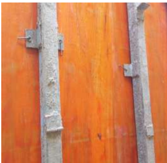
(a) Nailing to plywood
