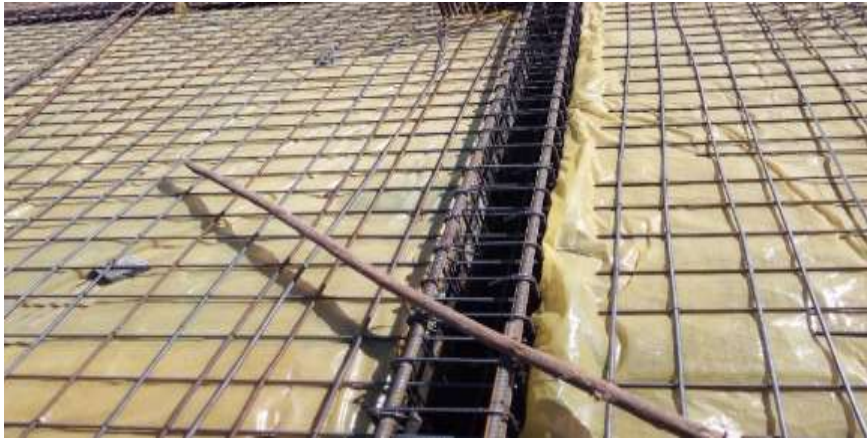
Figure 4. 7 Thin plastic sheets applied over plywood to protect paste
