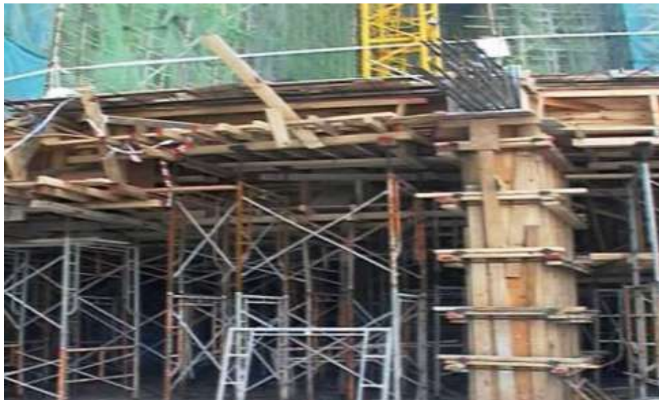
Figure 2.8, Modern conventional formwork in building construction
