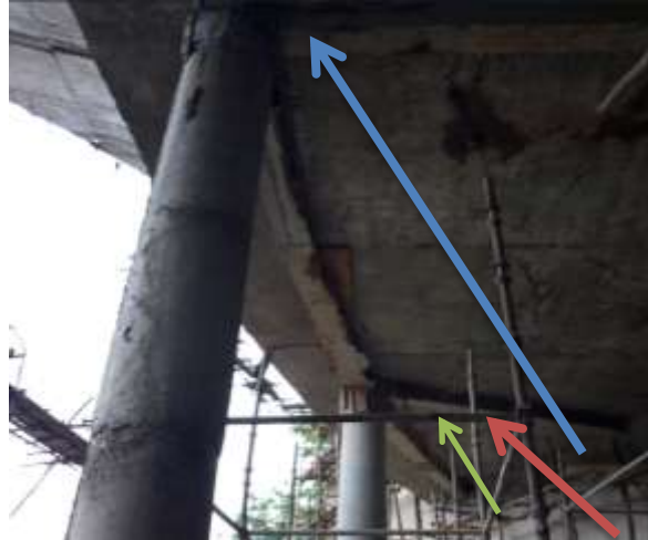
(d) poor finishing/ pieces of forms bonded on surface
