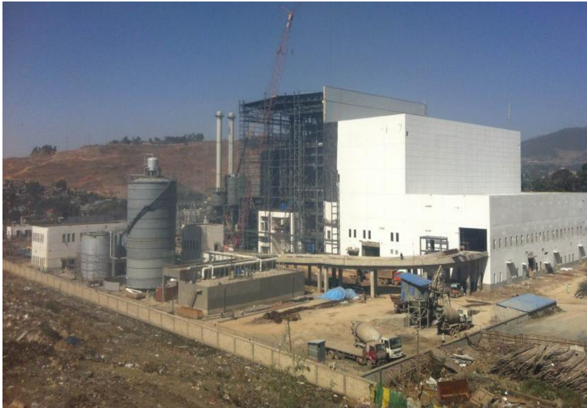
Figure 1. The construction site of Reppi (AACA)
