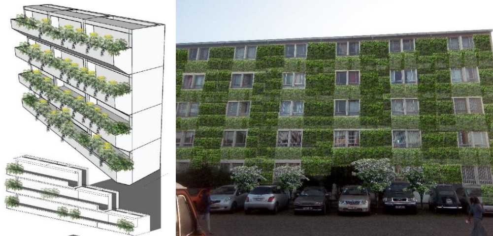
Fig 59: New construction of living wall, (Source: Author)
