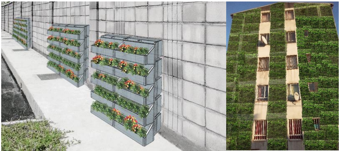
Fig. 58: Construction of green wall over bare walls, (Source: Author)
