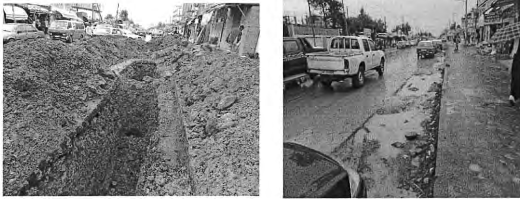
Figure 4.2 picture showing excavation of roads within the carriage of way
