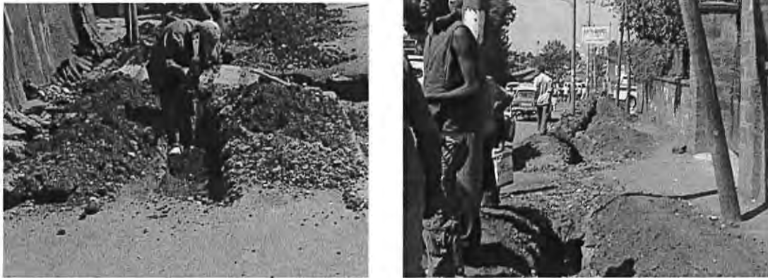
Figure 4.4 picture showing excavation of roads using “Doma” in the inner city
